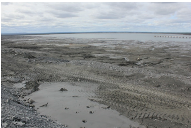
Fig. 2. Tailing dump «Lebyazhe», Norilsk industrial region (photo by Grebenets V.I., August 2018).
